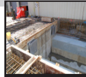
1 Reaction Mass Footings
